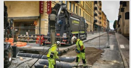
*Simple operation, less back-breaking work, and excavating cables without causing damage – RSP suction excavators takes the weight out of many civil engineering jobs.*
